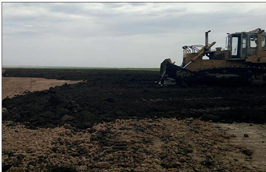
Figure 5. Applying a peat-sand mixture with a bulldozer
