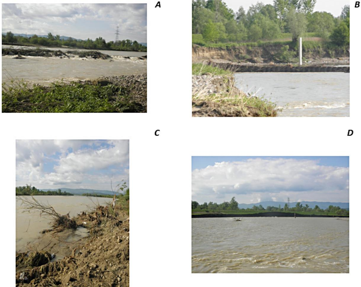
**Figure 1.** Photographic documentation of the damage to the area of the surface intake on the Dunajec River in Świniarsko in 2014: branches and rubble deposited by the flood wave (A); damage to the river banks (B-C); damage to the flood embankment on the other side of the intake (D) [WTP archive]
