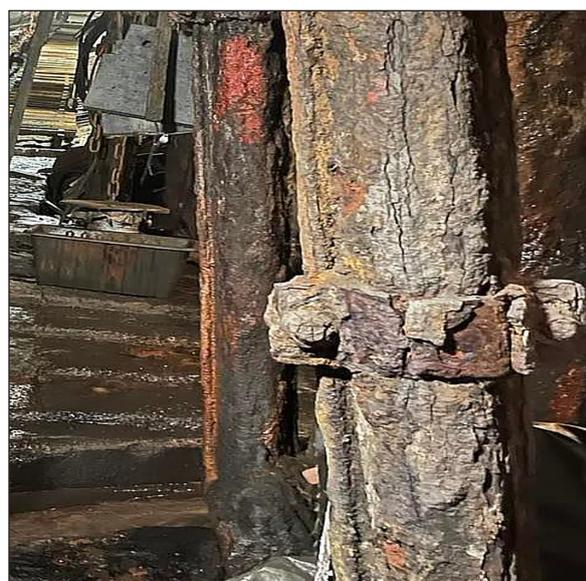
**Fig. 7.** Corrosion cracking in a moist environment, accelerated by stresses in the material. The vicinity of the shaft's riser 1.3 (Photo: M. Ciosmak)
