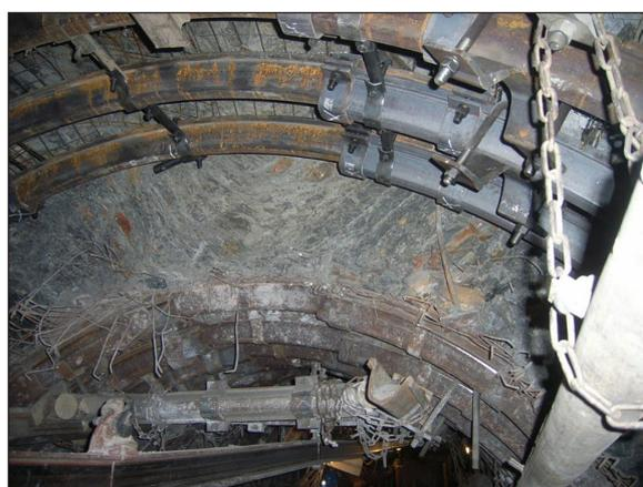
Fig. 5. Replacement of support due to tightening (convergence) as a result of the impact of the rock mass surrounding the excavation (Source: Wiadomości Górnicze Nr 3/2016)
