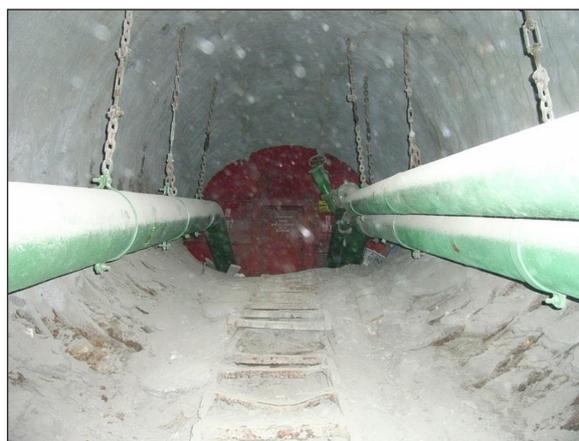
Fig. 4. DN400 main drainage pipelines and mine excavations with visible sprayed concrete
