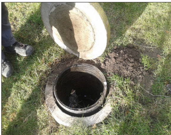
Figure 6. Condition of a manhole
