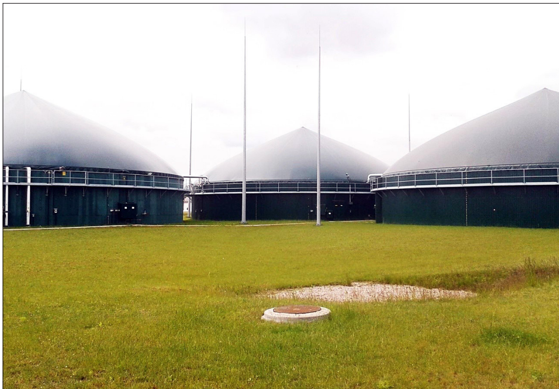
Fig. 2. Adler Biogas power plant
