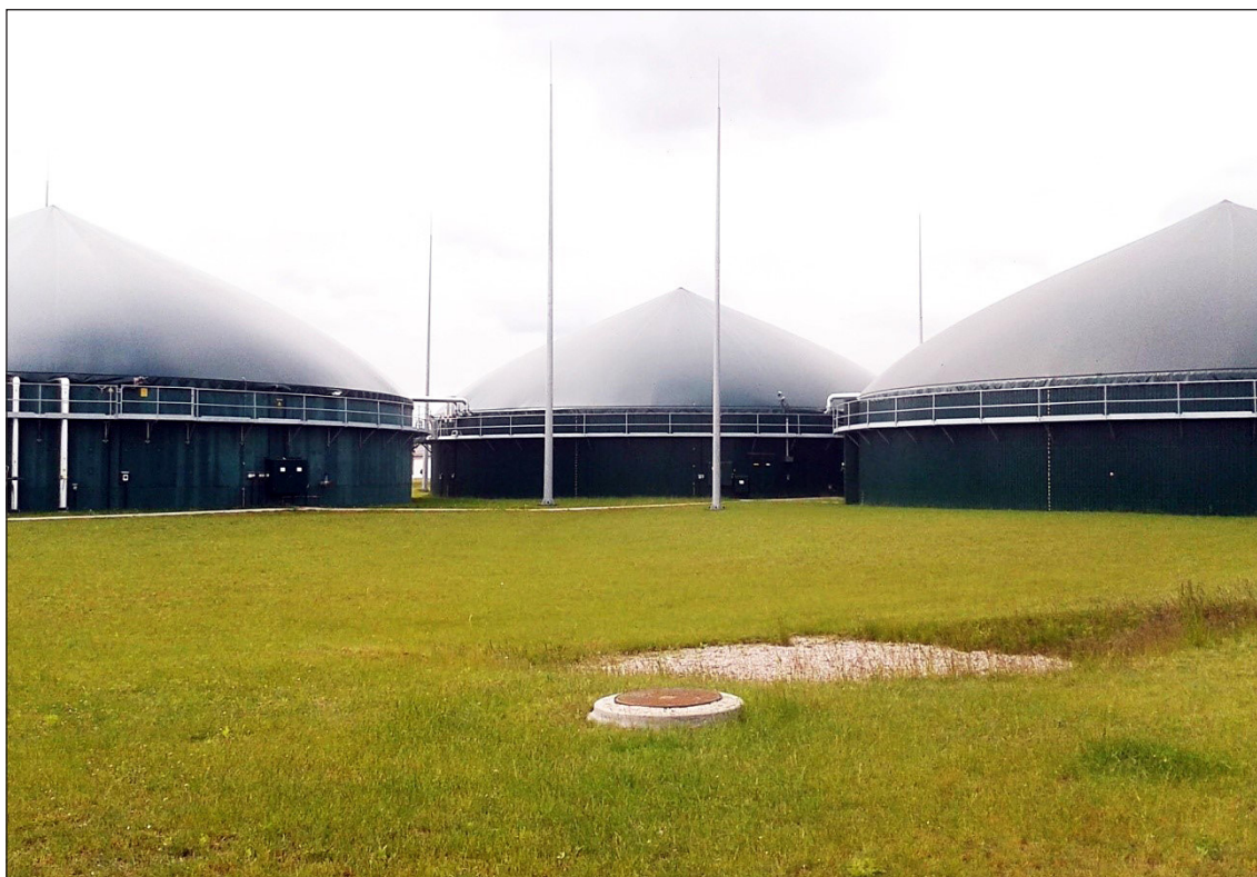
Fig. 2. Adler Biogas power plant
