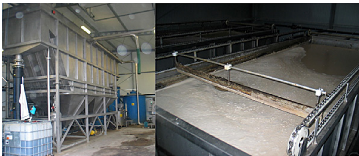
Figure 1. DAF flotation in Bielmlek WWTP
