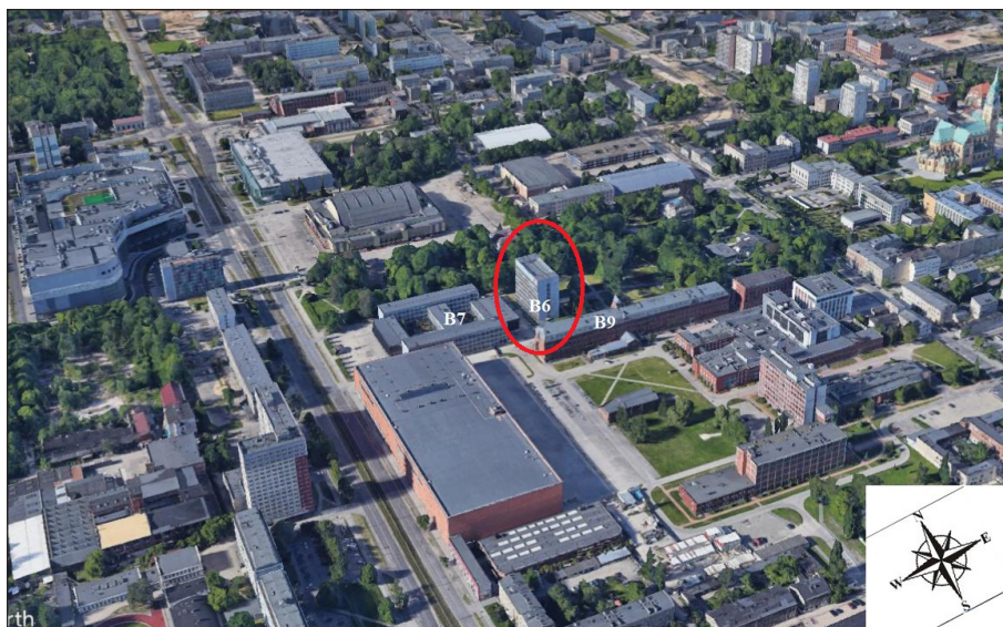
Fig. 1. Location and surroundings of building “B6” on campus “B” of Lodz University of Technology (photo source: www.google.com/maps )
