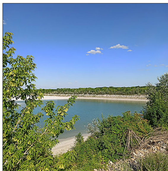
Figure 1. Photo of the alkaline lake of sludge storage No. 4
