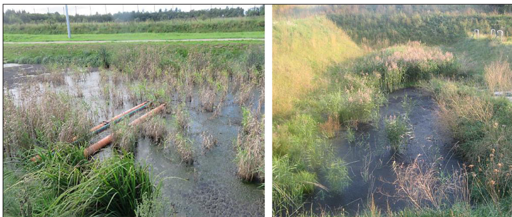
Figure 2. STRB in Gniewino, which experienced operational problems in 2017 (photo: Gniewino WWTP, Dariusz Rohde)
