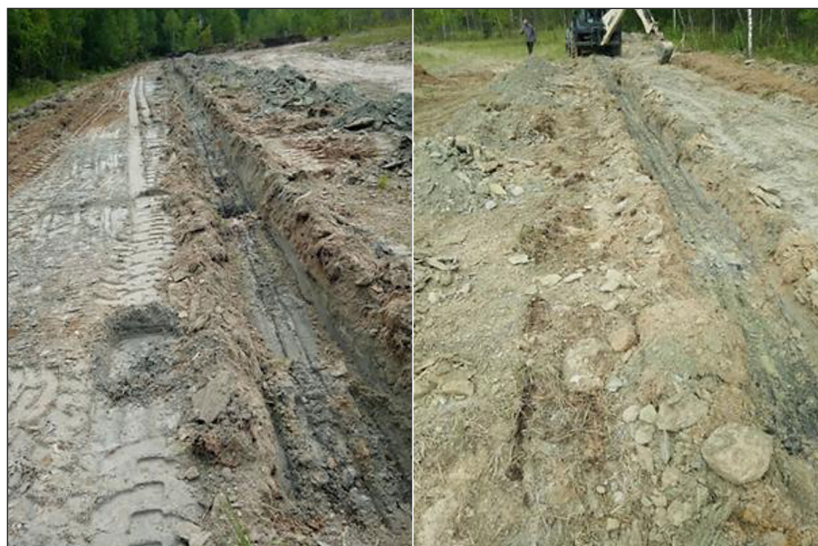
Figure 4. Construction of depressions to create the necessary soil layer thickness at tree planting locations
