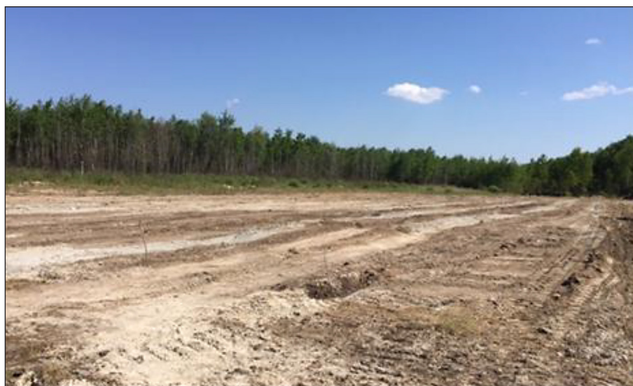
Figure 3. Results of surface leveling and filling subsidence areas of part of the tailings storage facility territory
