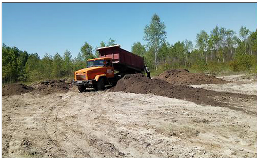
Figure 5. Surface coverage of reclamation with a fertile soil layer
