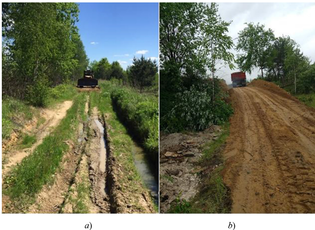
Figure 2. Construction of road through tailings storage facility dam to enable engineering equipment access to work site: a – initial stage of equipment work, b – engineering equipment passage
