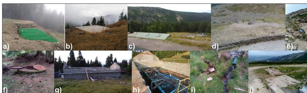
Figure 5. Components of the mountain water and wastewater management system in the Karkonosze National Park: a-d) unprotected sediment tank, e-f) unprotected element of water supplying system, g-h) unprotected wastewater treatment plant building, i) discharge untreated wastewater to receiver, j) unprotected subsurface leaching system, photo: Pawęska/Dąbek, 2018–2019
