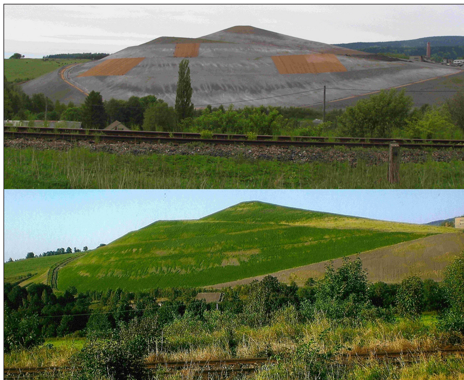
Figure 2. Reclamation of the central mine waste dump (photo by A. Grmela)
