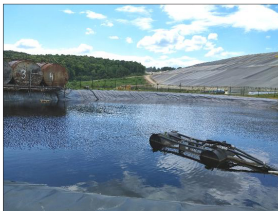
Figure 2. New leachate collection reservoirs at the Lviv MSW landfill
