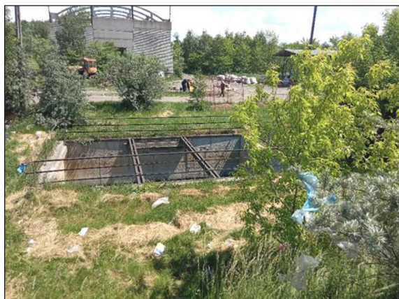
Figure 3. General view of the leachate collection tank at the Chervonohrad MSW landfill
