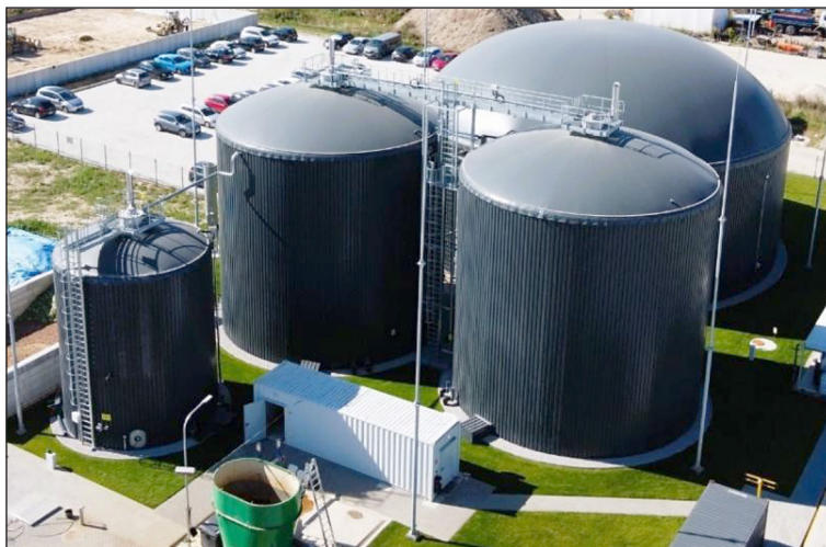
Figure 2. Full-scale agricultural biogas plant (0.499 MW) with a dedicated acid hydrolysis stage
