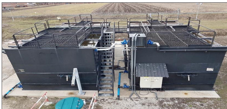
Figure 2. Conventional activated sludge tank reactor
