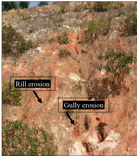
Figure 4. Rill and gully erosions observed at the study area
