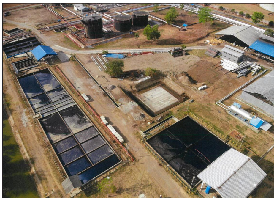
Figure 1. Main gathering station wastewater treatment plant of Balongan
